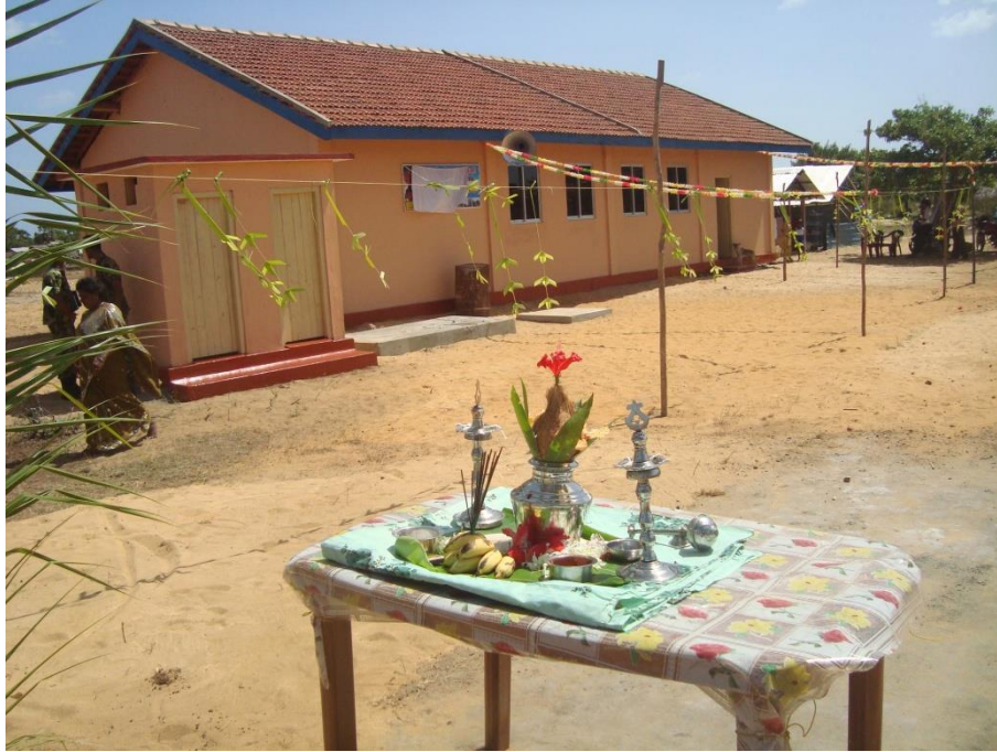
Chandran Pre-School in Mullivaikal East after Rebuild/Renovation in June 2013
