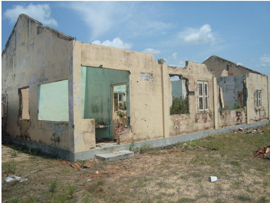
Chandran Pre-School in Mullivaikal East before Rebuild/Renovation
