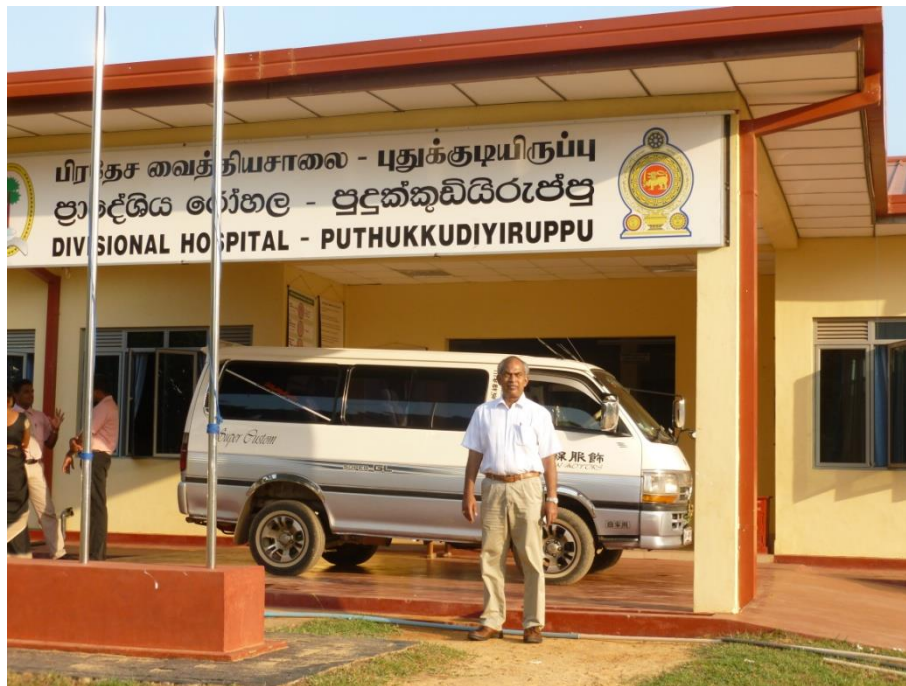
Recently built main building of the hospital
