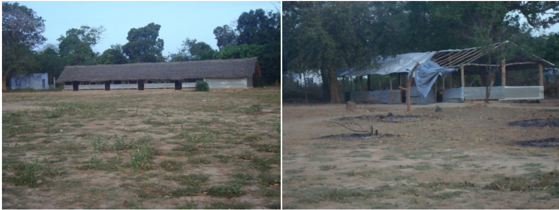
Photos 5&6: Temporary buildings available in the school seen in June 2013
