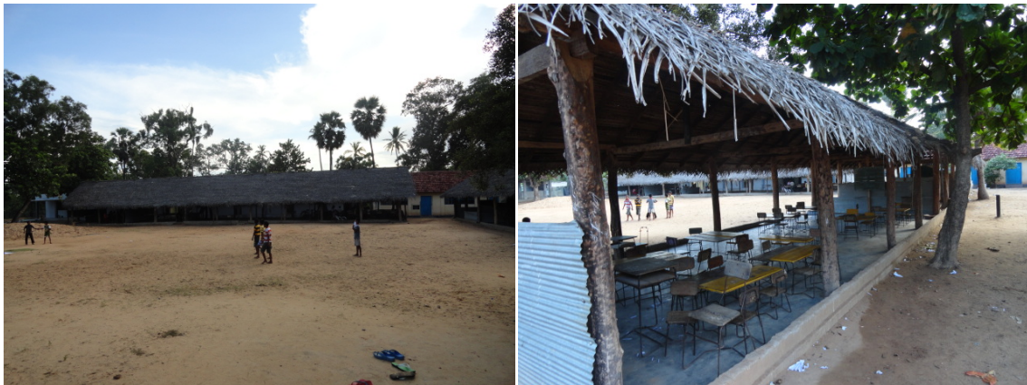
Photos 15&16: Two temporary functioning shelters at Iranaippalai GTM School
