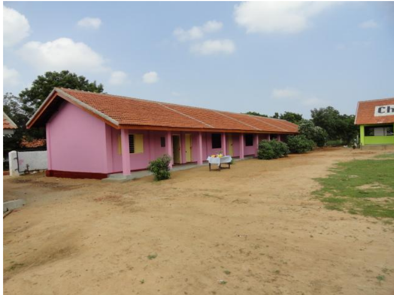
Renovated building was re-opened on 17 Jan 2014
