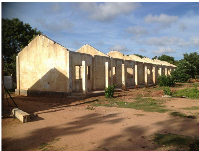
Before Renovation work of the building that was being repaired
